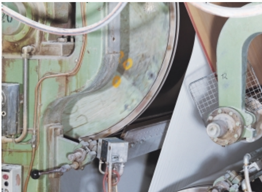
◀ The robust design and large scanning distance are of advantage to the WT 45 photoelectric proximity switch when used to check for tear-off on a paper rolling machine.
